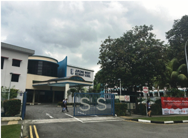
Jurong West Secondary School Electrical Works - Completed 2001
