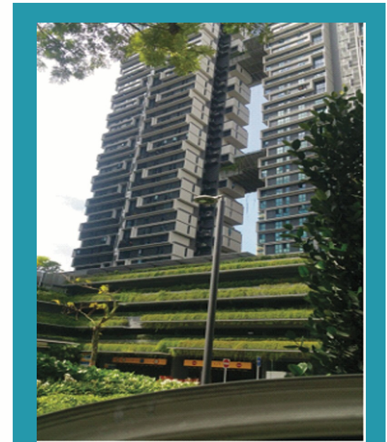
Dawson Contract 2 Electrical Works - Completed 2015
