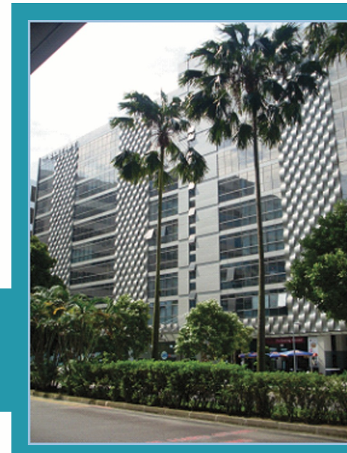
The Elitist @ Bukit Batok Crescent Electrical Works – Completed 2013
