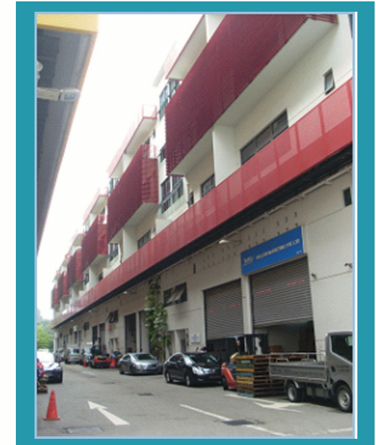
The Splendour @ Bukit Batok Crescent Electrical Works & Lift Installation – Completed 2012
