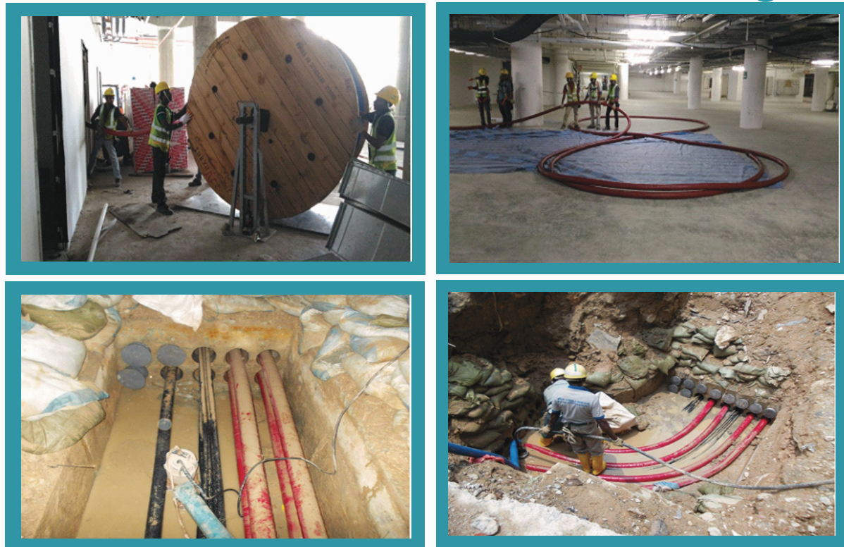
Underground HT / LT Cabling Works
