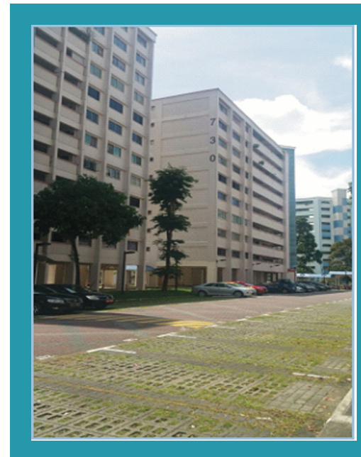
Upgrading Project for G146F, Yishun Electrical Works - Completed 2015
