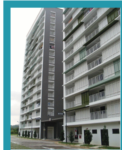
N8C32C @ Tampines Street 86 Electrical Works & Escalator Installation - Completed 2016
