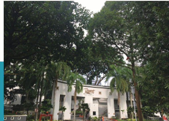
Regent Height Condominium Electrical Works – Completed 1997
