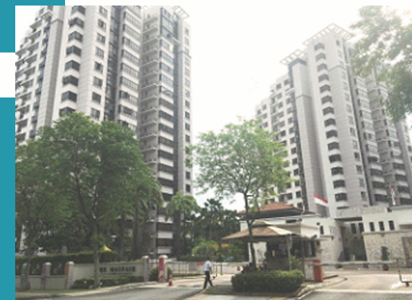
Mayfair Condominium Electrical Works – Completed 1999
