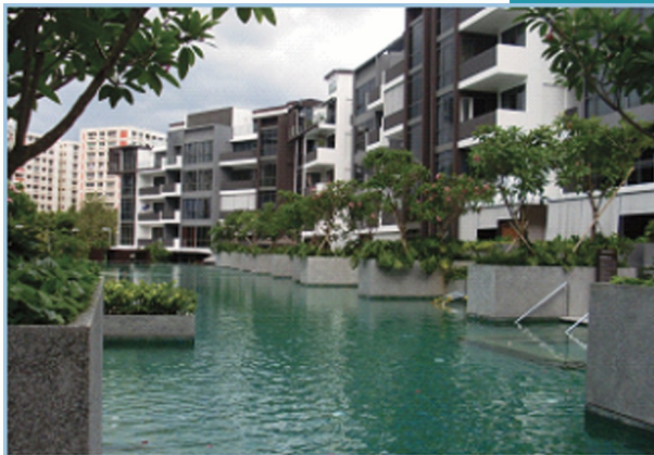
Stratum @ Pasir Ris Drive Electrical Works & Platform Lift Installation – Completed 2016
