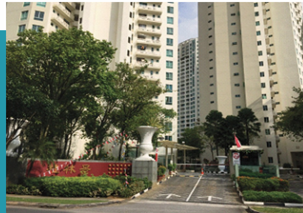
Guilin View Condominium Electrical Works – Completed 1998
