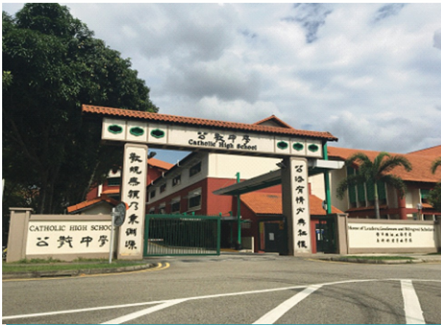
Catholic High School Electrical Works - Completed 2004
