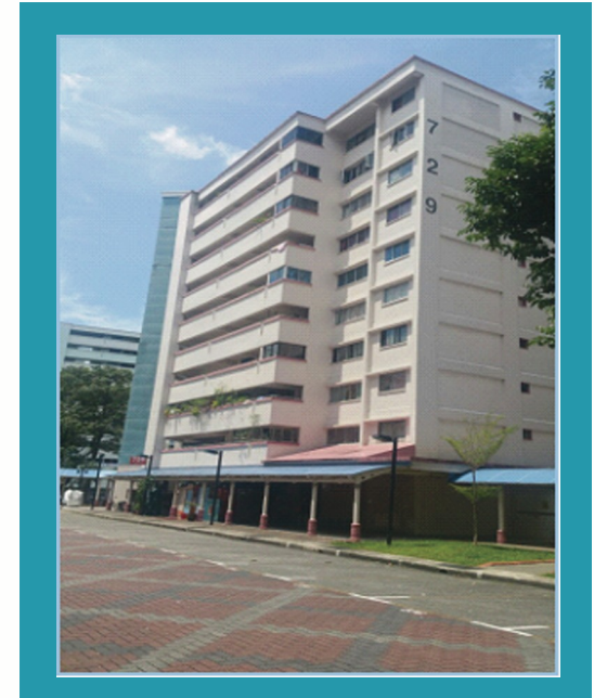
Upgrading Project for G146F, Yishun Electrical Works - Completed 2015
