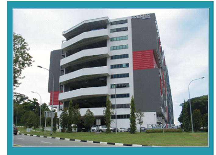
Premier @ Kaki Bukit Electrical Works – Completed 2014
