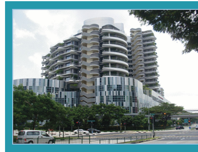
Jurong Community Hospital (Ng Teng Fong Hospital) Data & Fibre Cabling Works – Completed 2014
