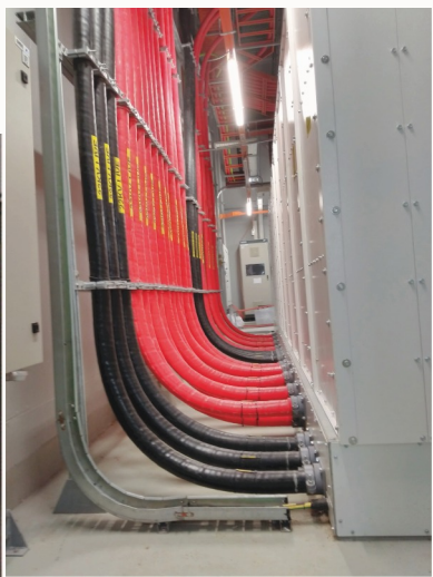
Micron Fab 10 Extention (Fab 10X) F11D High Tension Switchgear and Cabling
